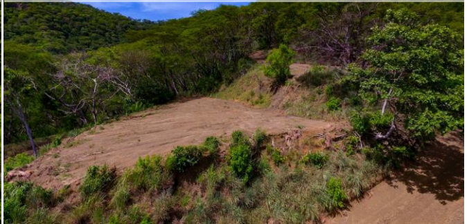
Lower Level Building Pad
